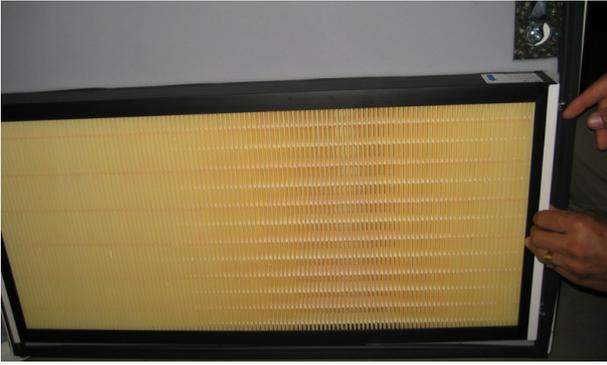
On a Airmaster 900, the exhaust air filter is either fitted at the top (displacement ventilation) or the bottom (mixing ventilation) of the front cover.
