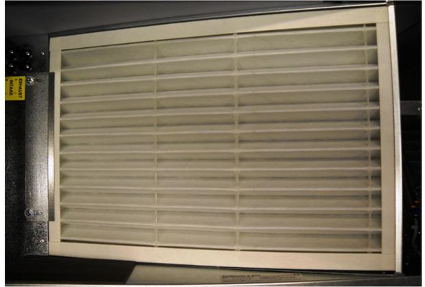
5. The support plate for the fresh air filter is under the exhaust air filter:
