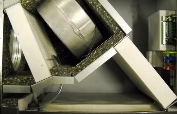
2. Filters without support plate (on the left) and with support plate (in the centre of the illustration):
