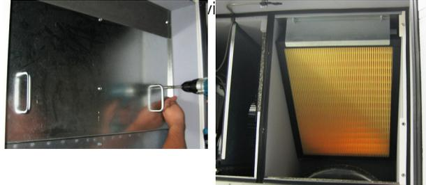
At the top of the unit, the filter is fitted in a support plate behind a service cover.
