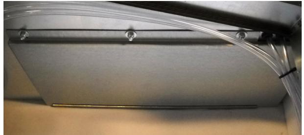
On some models the exhaust air filter is fitted using a support plate. Under the filter, a guard is fitted for the fresh air filter. Here the fresh air filter consists of two filter elements.
