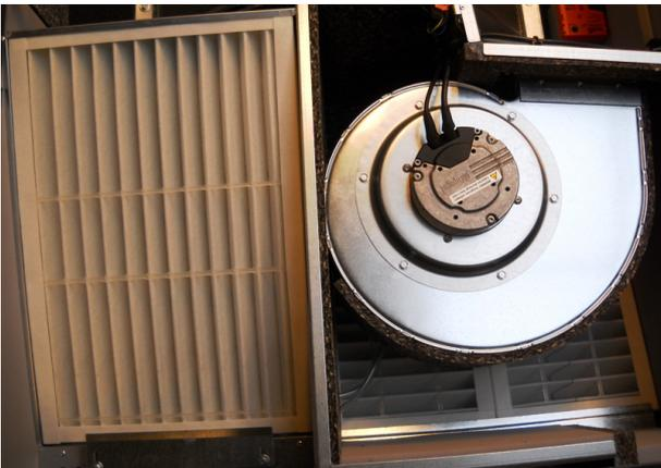
4. Exhaust air filter with support plate:
